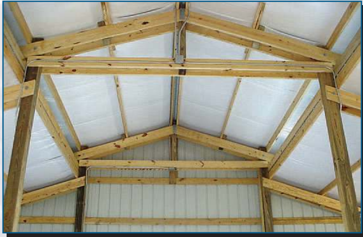
Wood Purlin on Wood Truss
